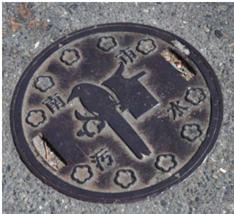
Manhole Cover in Tainan
